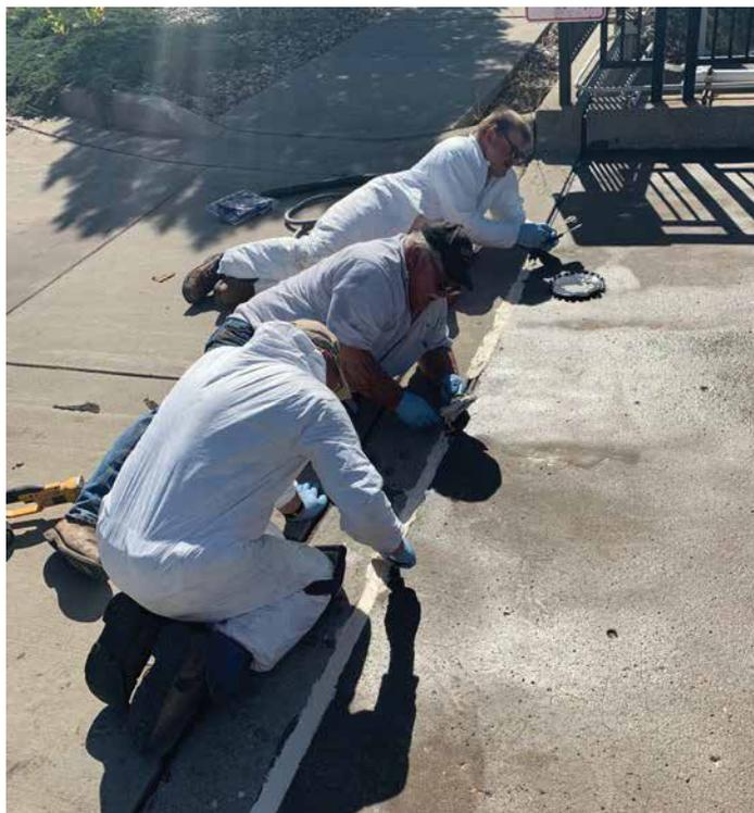
Resealing expansion joints and concrete deck maintenance activities at the Snake Creek Pumping Plant.
