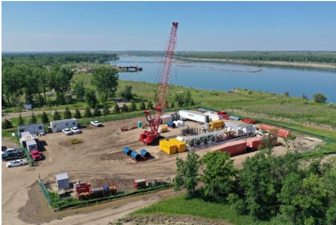
Site Under Construction
