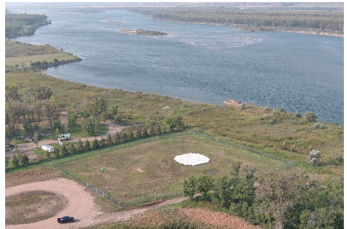
Completed Missouri River Intake
