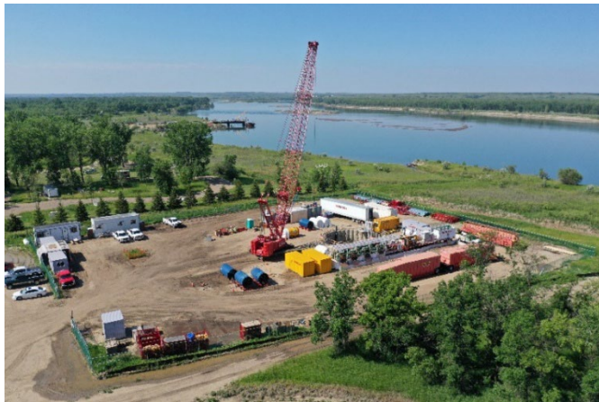
Site Under Construction
