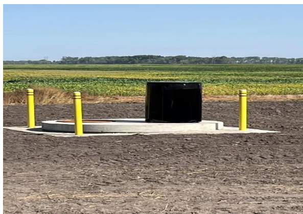
Typical Air Release Manhole
