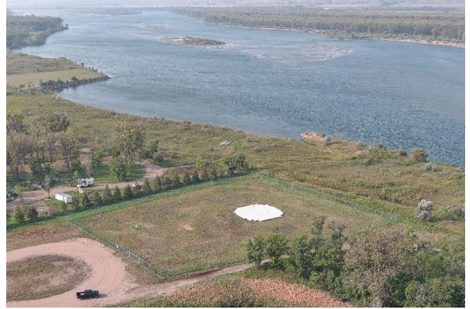
Completed Missouri River Intake
