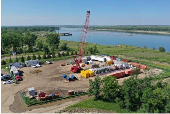
Site Under Construction
