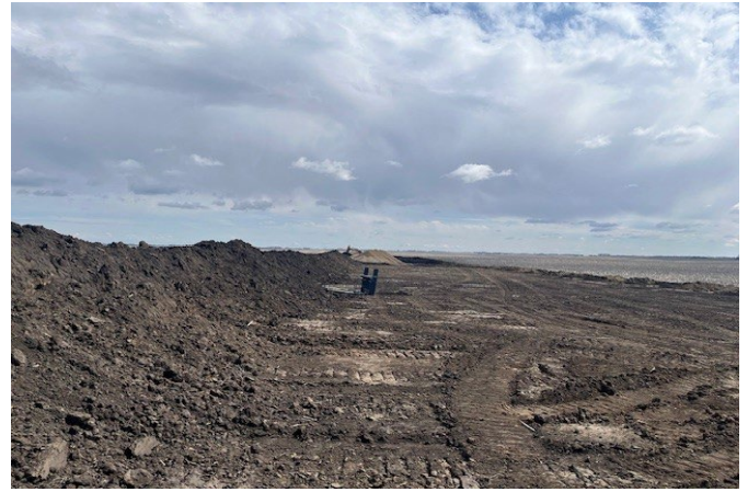
Topsoil Removal
