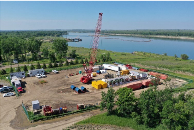
Site Under Construction
