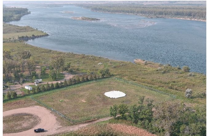
Completed Missouri River Intake
