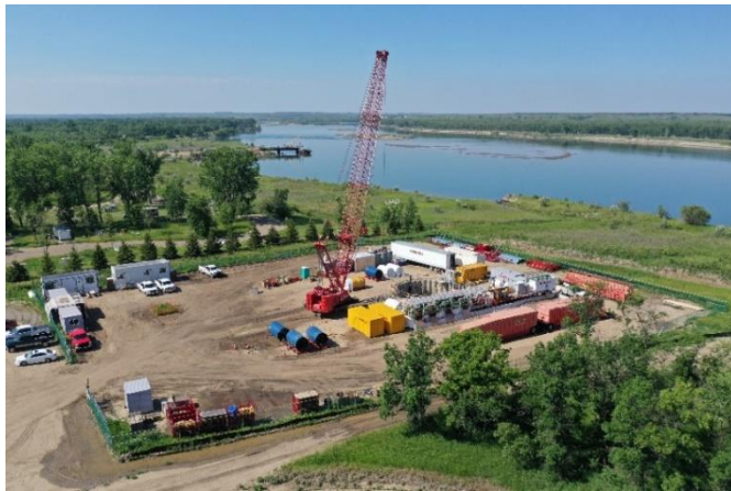
Site Under Construction
