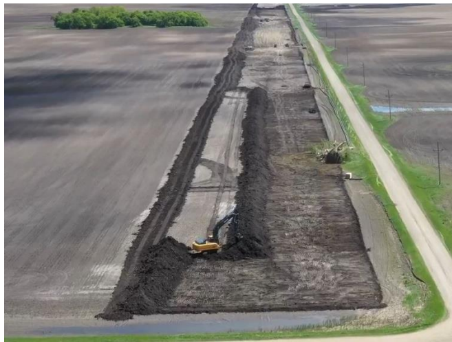
Stripping Topsoil
