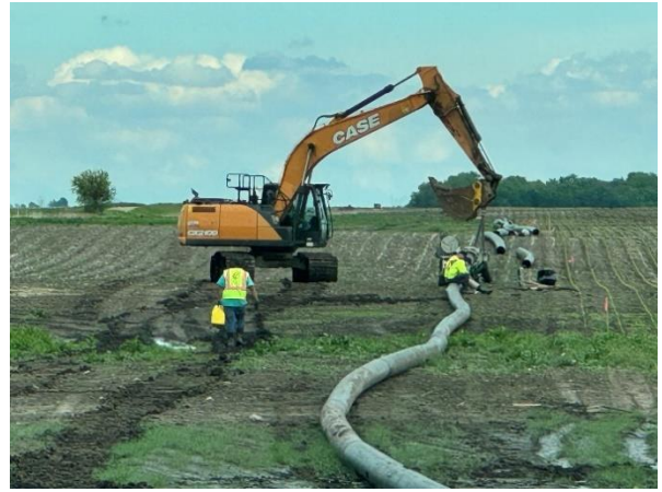
Placing Dewatering Pipe
