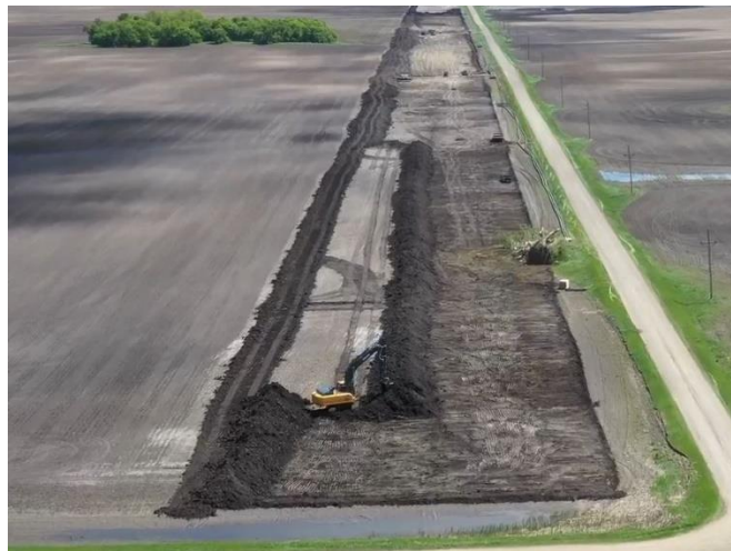
Stripping Topsoil
