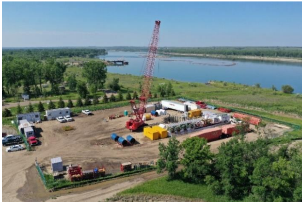
Site Under Construction
