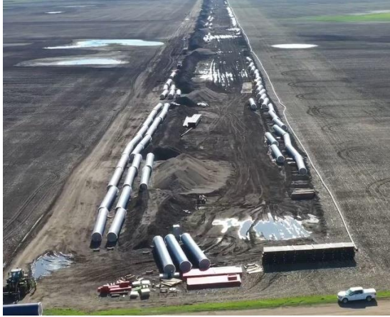
Stored Pipe on Site
