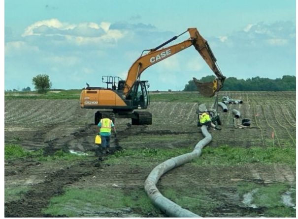
Placing Dewatering Pipe
