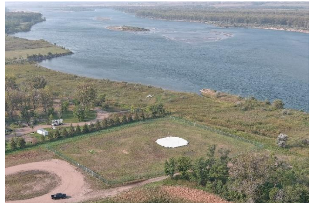
Completed Missouri River Intake
