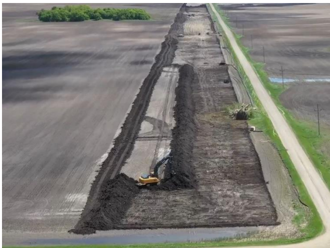
Stripping Topsoil
