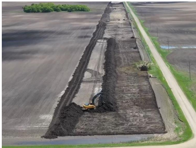
Stripping Topsoil
