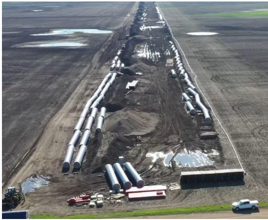
Stored Pipe on Site
