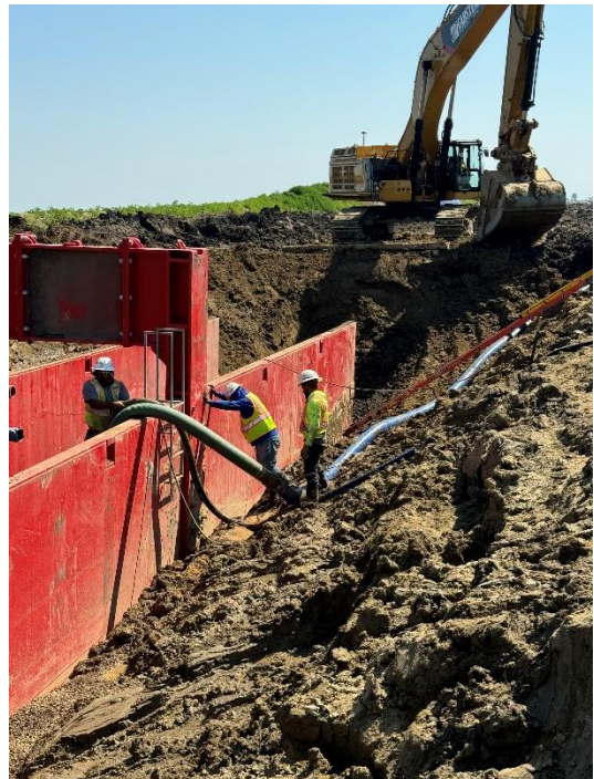
Trench Box w/ Dewatering Pipes
