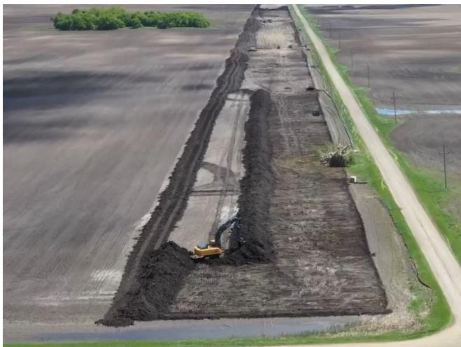
Stripping Topsoil
