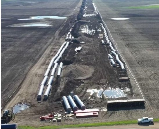
Stored Pipe on Site
