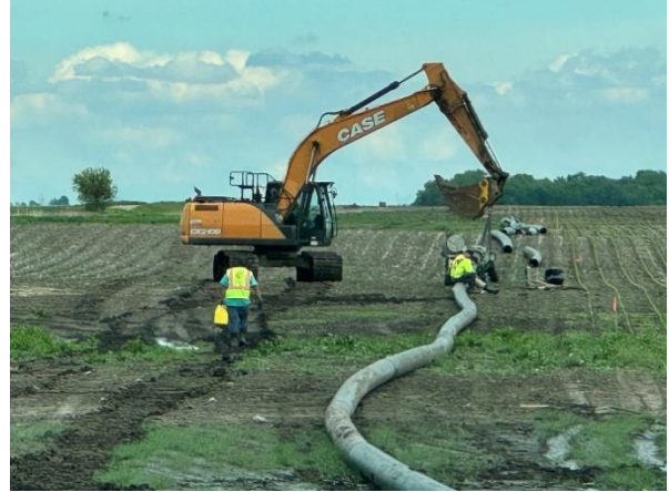
Placing Dewatering Pipe
