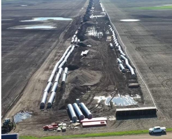
Stored Pipe on Site
