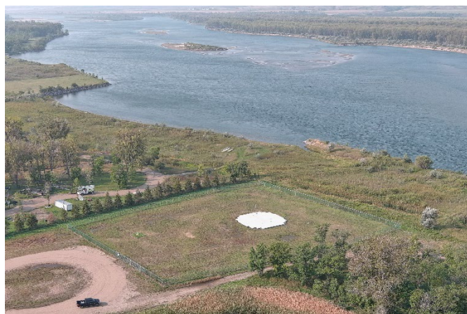
Completed Missouri River Intake
