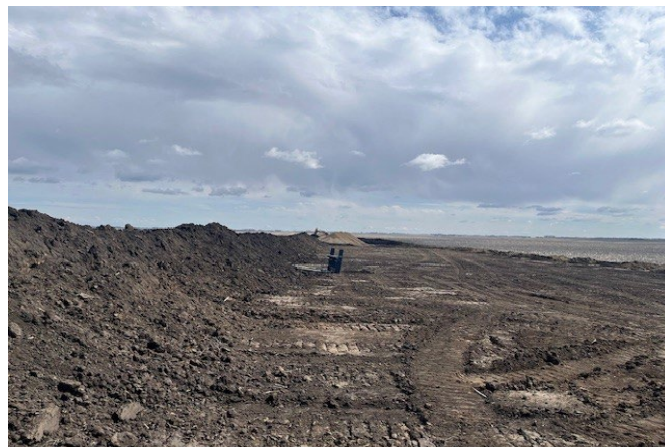
Topsoil Removal
