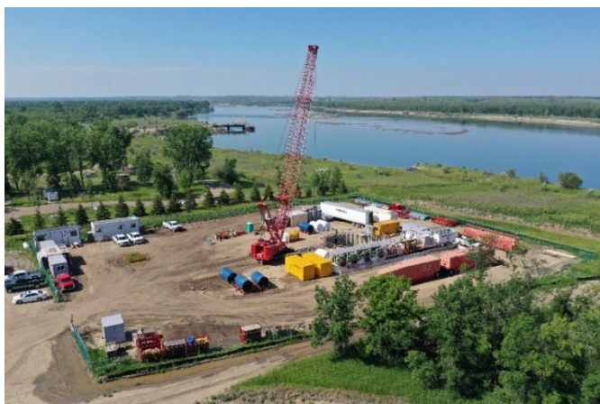
Site Under Construction
