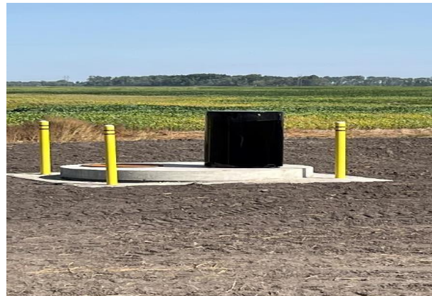
Typical Air Release Manhole
