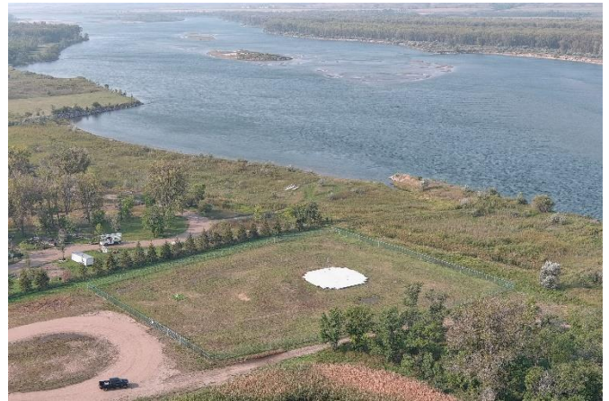
Completed Missouri River Intake
