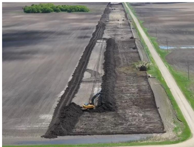
Stripping Topsoil
