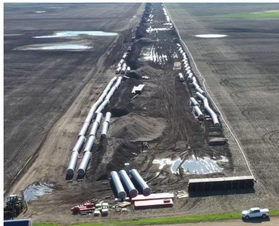
Stored Pipe on Site
