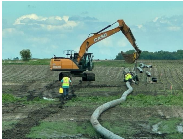
Placing Dewatering Pipe
