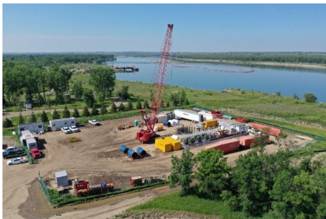
Site Under Construction
