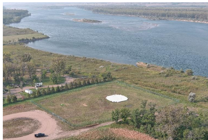
Completed Missouri River Intake
