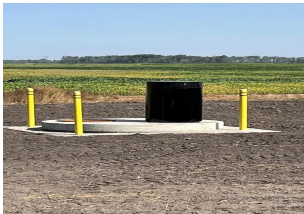
Typical Air Release Manhole
