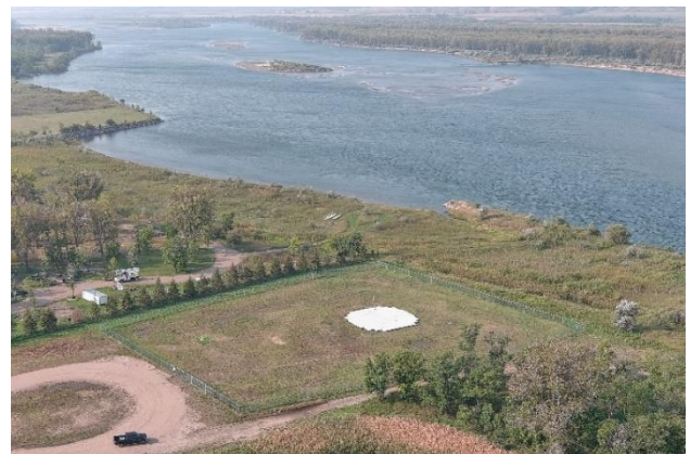
Completed Missouri River Intake
