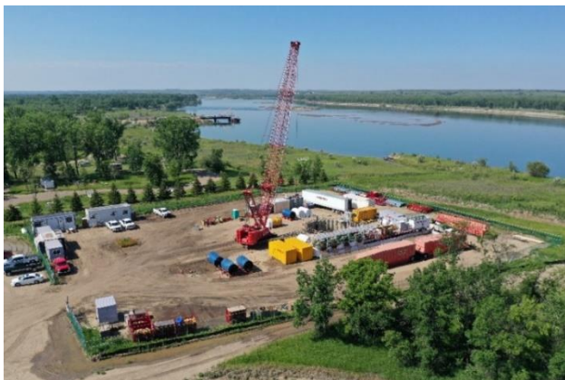
Site Under Construction
