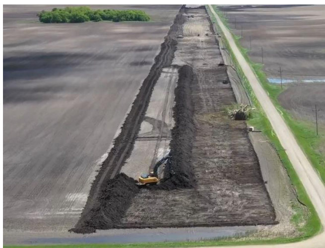
Stripping Topsoil
