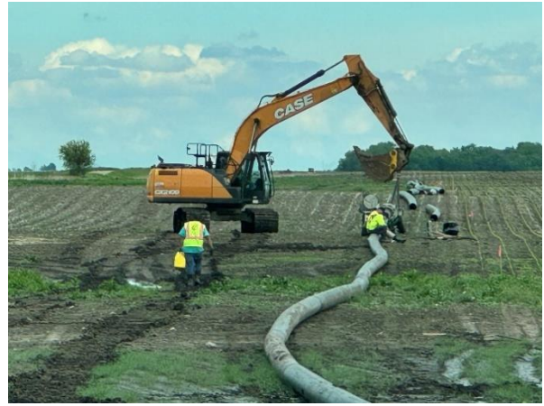
Placing Dewatering Pipe
