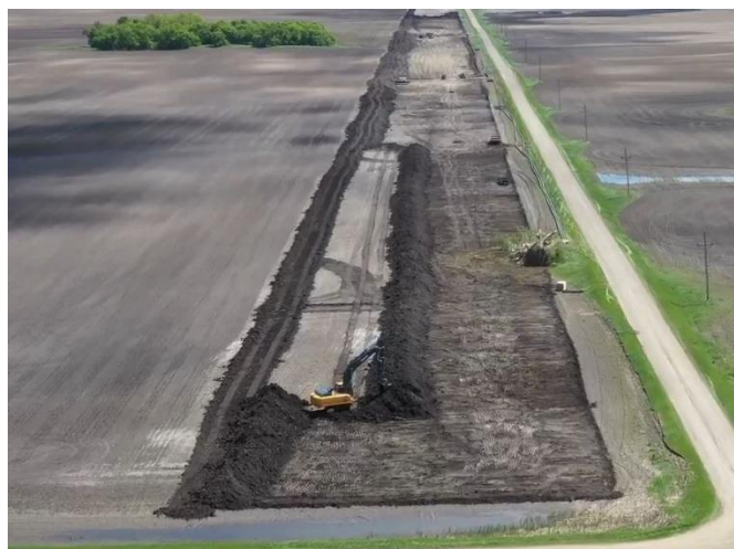
Stripping Topsoil
