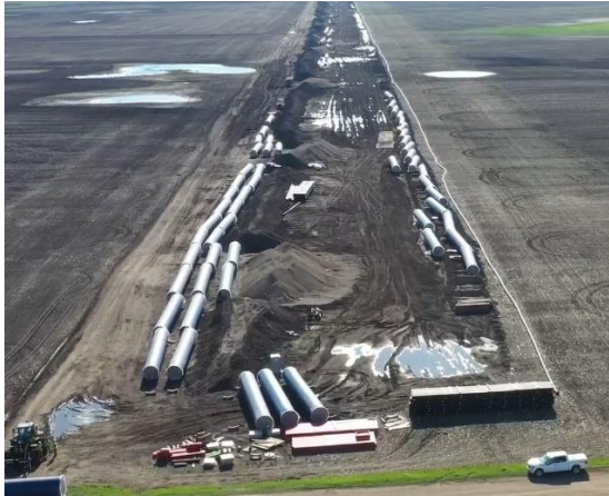
Stored Pipe on Site
