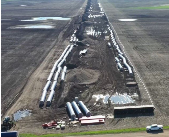
Stored Pipe on Site
