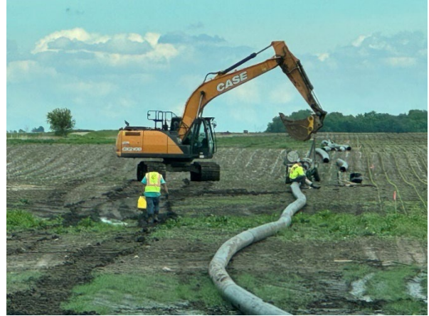
Placing Dewatering Pipe
