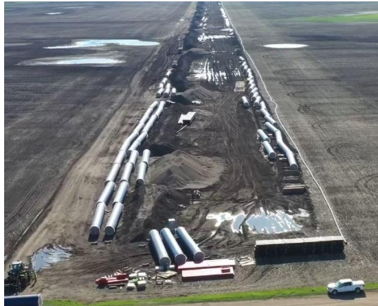
Stored Pipe on Site
