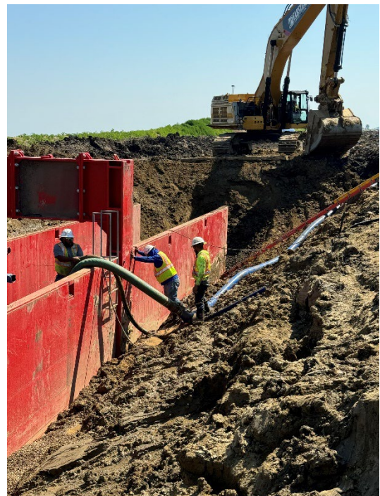
Trench Box w/ Dewatering Pipes
