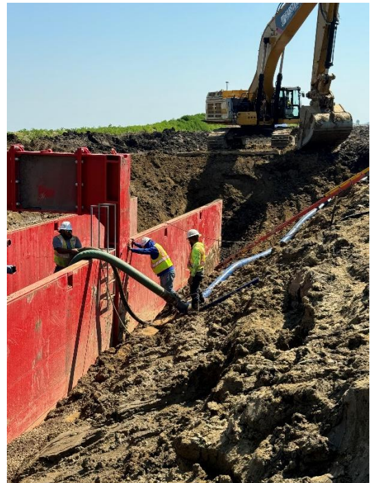
Trench Box w/ Dewatering Pipes
