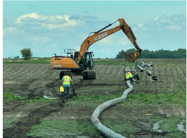
Placing Dewatering Pipe
