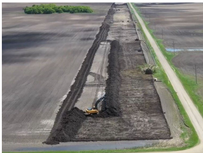
Stripping Topsoil
