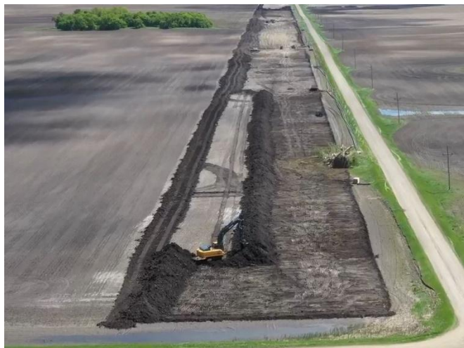
Stripping Topsoil
