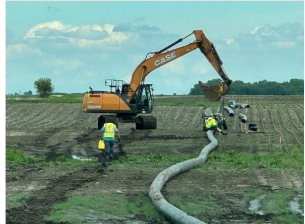
Placing Dewatering Pipe
