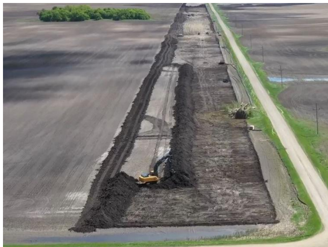
Stripping Topsoil
