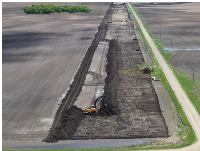
Stripping Topsoil
