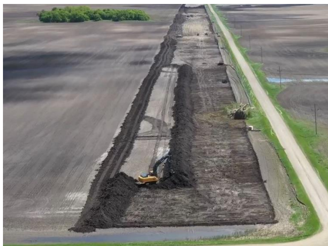
Stripping Topsoil
