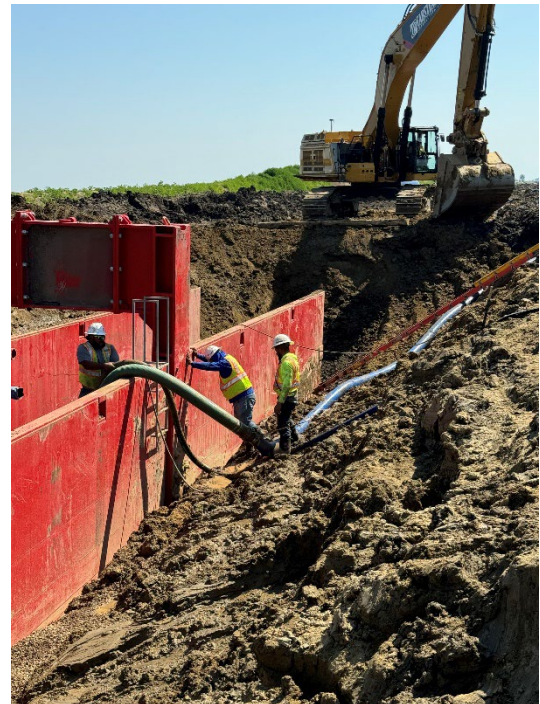
Trench Box w/ Dewatering Pipes
