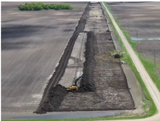
Stripping Topsoil
