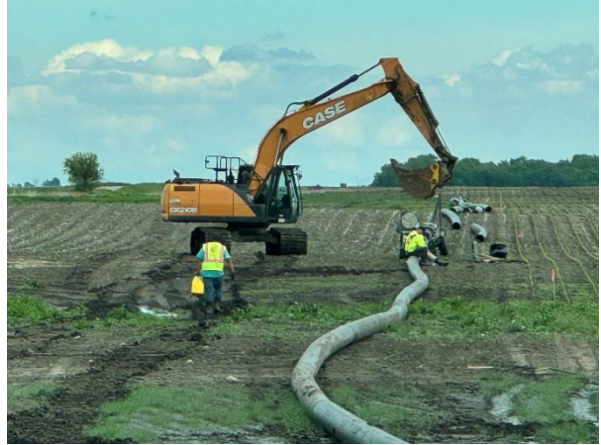
Placing Dewatering Pipe
