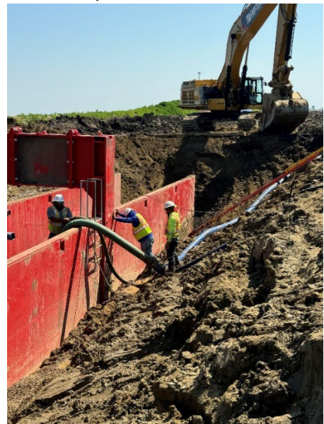
Trench Box w/ Dewatering Pipes
