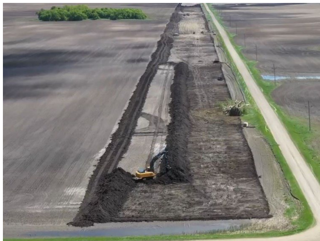
Stripping Topsoil
