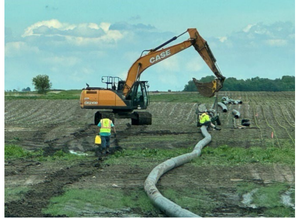
Placing Dewatering Pipe
