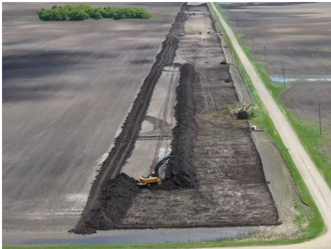
Stripping Topsoil
