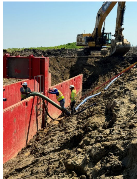
Trench Box w/ Dewatering Pipes
