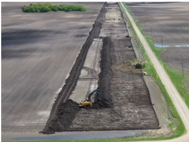
Stripping Topsoil
