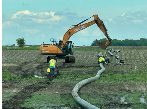
Placing Dewatering Pipe
