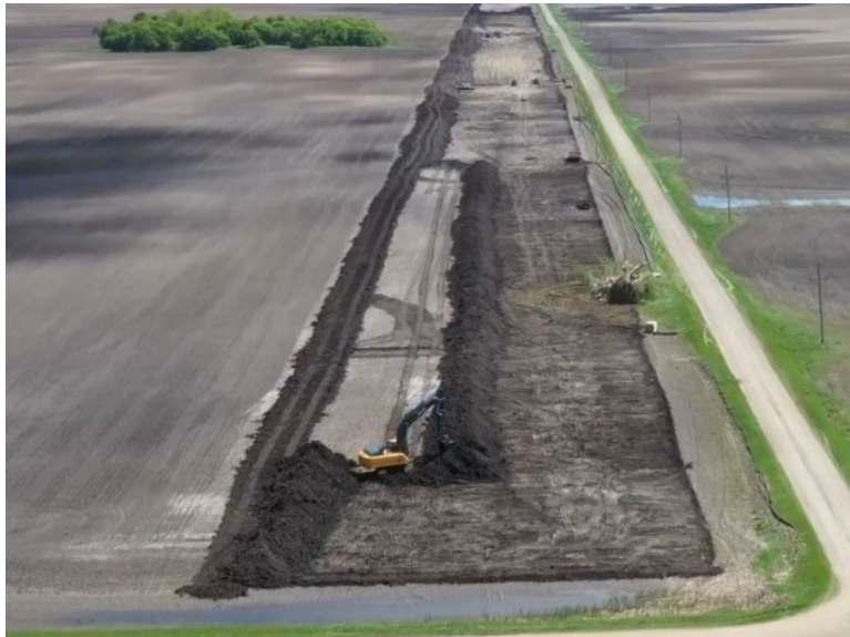
Stripping Topsoil
