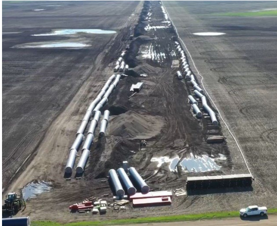
Stored Pipe on Site
