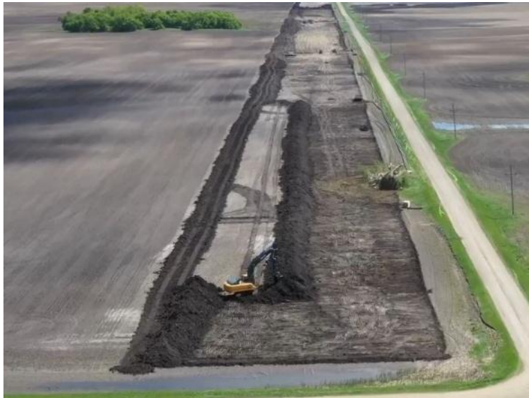
Stripping Topsoil
