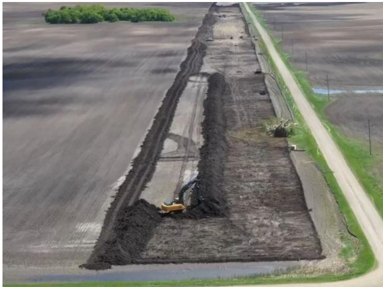
Stripping Topsoil
