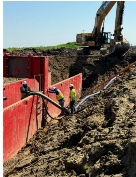
Trench Box w/ Dewatering Pipes
