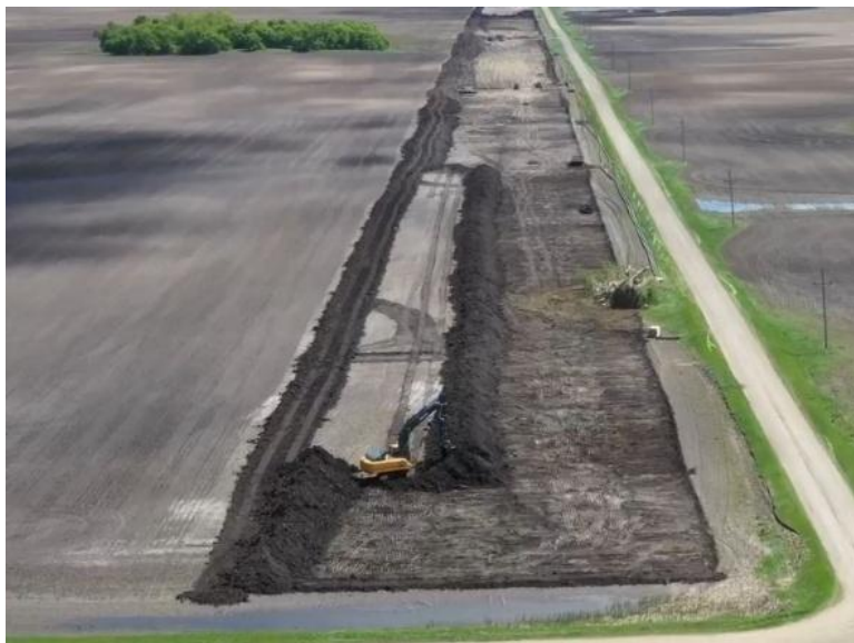
Stripping Topsoil
