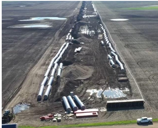
Stored Pipe on Site
